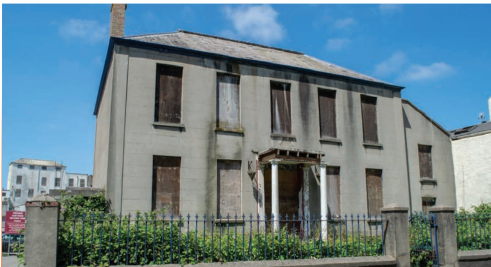
Sans Souci, St Saviours Road , owned by Andium Homes. Part of a large development site based on the former Ann Street Brewery, listed building Grade 3. A substantial, high-quality house built in the 1820s, vacant and boarded up for many years and awaiting redevelopment.*
