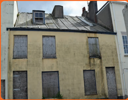
Nos 4 and 4a Simon Place, St Helier owned by Andium Homes. Part of the former Ann street Brewery complex; listed buildings Grade 3. Almost certainly built and occupied by Elias Le Gros, Jersey's pre-eminent map maker of the 19th century, and later occupied by Hugh Godfray, a pupil of Le Gros and maker of the 1849 map of Jersey. Vacant and boarded for decades, partly stripped of its roof covering, and allowed to decay. Awaiting redevelopment.
