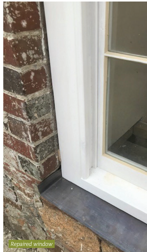
Before windows were repaired
