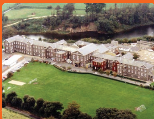
St Saviour's Hospital , owned by the States of Jersey. In the British Isles context, this is a rare and high quality example of a Victorian asylum, set in impressive landscaped grounds; listed building Grade 1. Substantially built and capable of conversion to new uses, this complex has been vacant and boarded up for many years.
